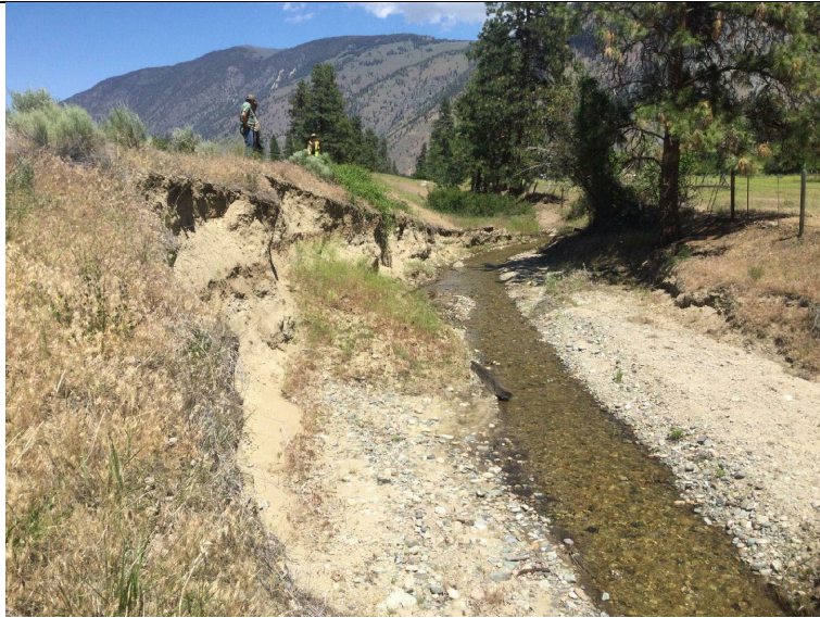
Photo 14: Downstream side of rail embankment (left) on Shoudy Creek showing high erosion and instability.
