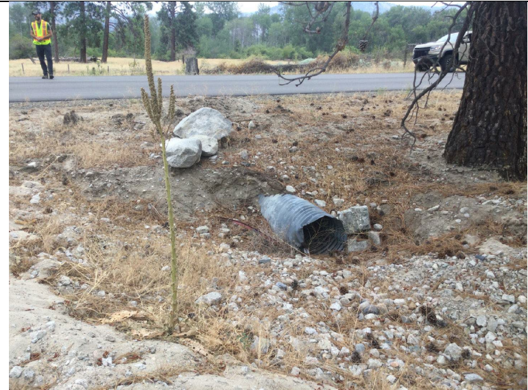
Photo 15: View of 600 mm diameter culvert at Chopaka Road along abandoned channel that was inundated during 2023 flood event.
