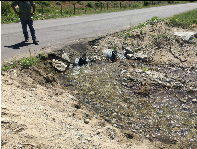
Photo 10: Current path of dominant flow (photo taken in June 2024). At 2023 washout location, inlet of two 600 mm diameter culverts on Chopaka Road.
