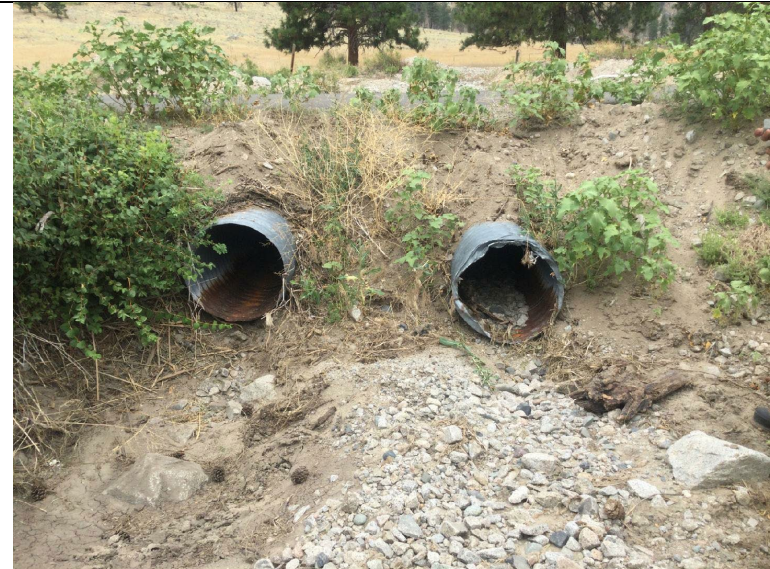
Photo 11: Outlet of two 600 mm diameter culverts on Chopaka Road.
