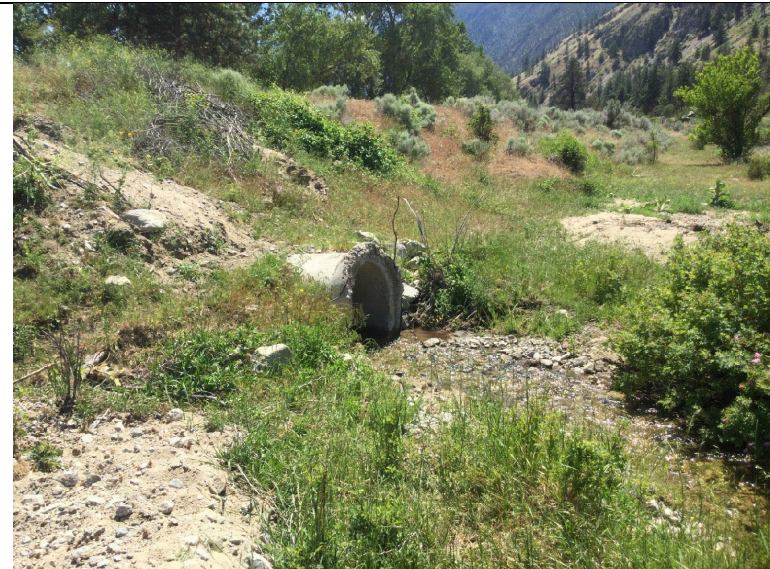
Photo 13: Immediately downstream from Chopaka Road, Shoudy Creek flows through a 900 mm diameter concrete culvert passing through old rail embankment.
