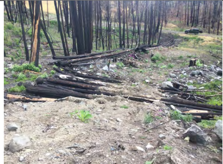
Photo 6: Corduroy stream crossing in area logged pre-wildfire (Red Bridge 1). Recommend rehabilitation of crossing due to anticipated increases in runoff.
