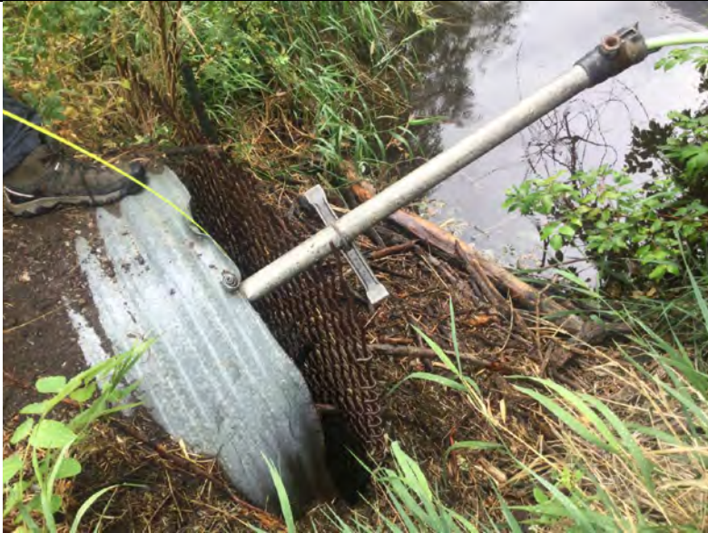
Photo 5: Culvert (4 ft (1220 mm) diam.) at Ashnola Road with upstream ponding associated with partial obstruction of flow.
