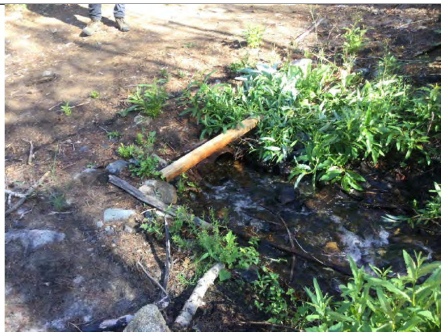
Photo 5: Webster Creek at Eart Creek Road, 500 mm diameter culvert is partly lugged with sediment. Ashnola River is 15 m downstream.
