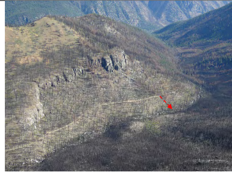
Photo 4: Section of Lakeview Road through steep canyon. Drainage-related landslide is indicated (arrow).
