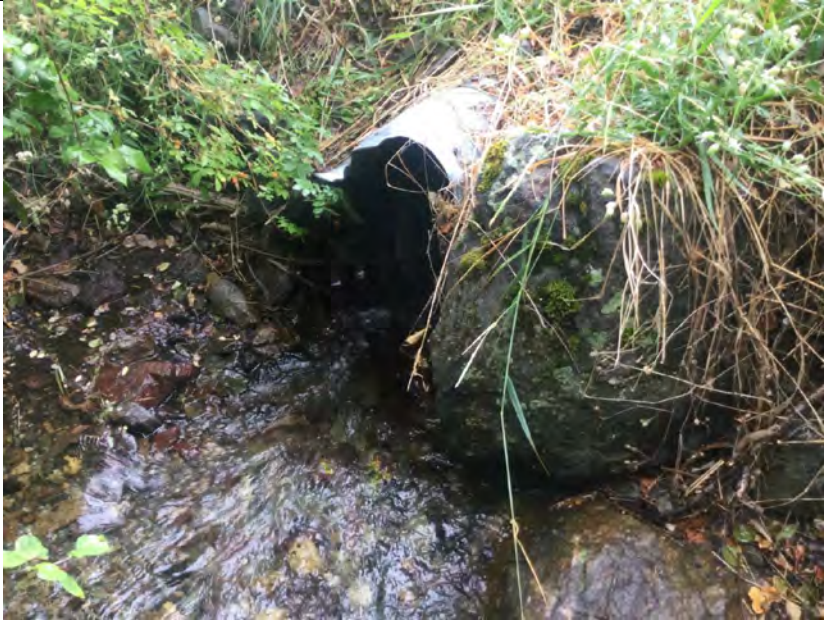
Photo 5: 600 mm diameter culvert at River Road, inlet damaged but free flowing. Some evidence of scour along streambanks but very little bedload movement.
