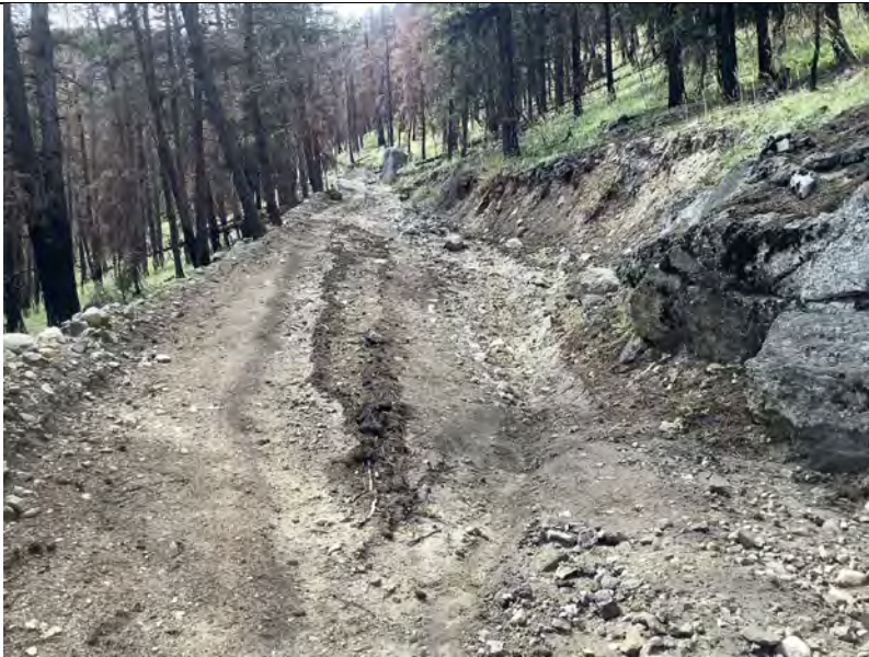
Photo 7: Example surface erosion associated with post-wildfire runoff onto Lakeview Road (~5.2 km).
