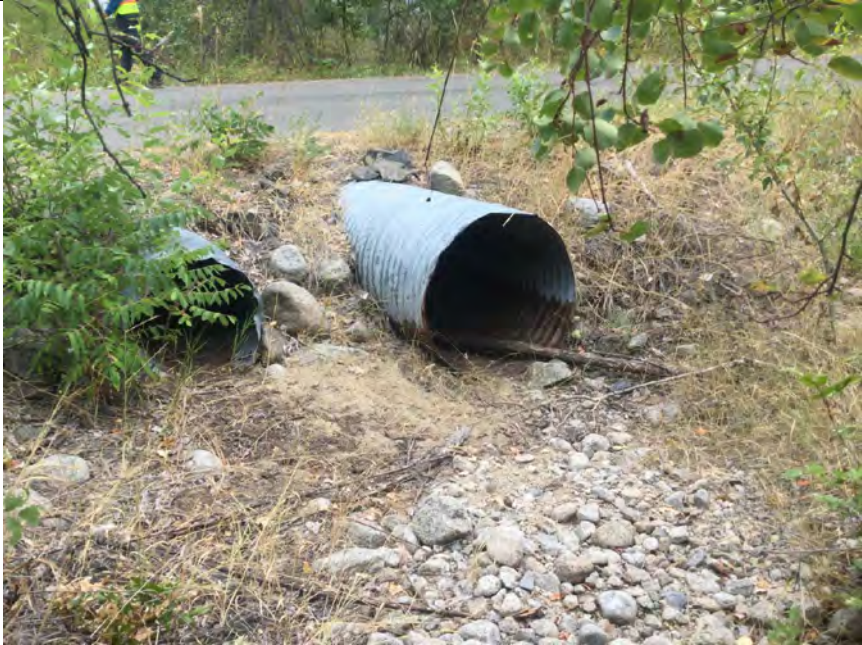
Photo 10: Two culverts on Chopaka Road at the seasonal channel in Photo 9 (600 mm and 800 mm diameter culverts).
