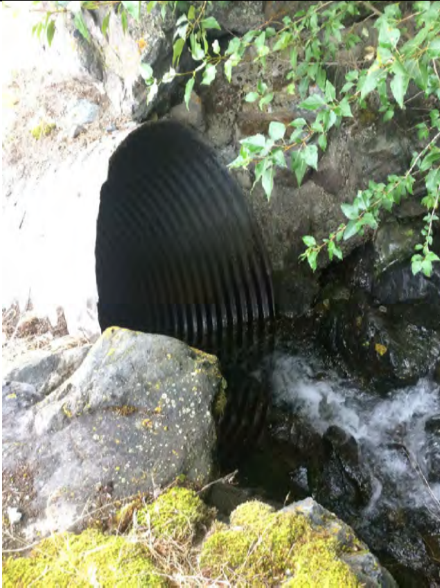
Photo 7: 5 ft (1,524 mm) diameter culvert encased in concrete at River Road is free flowing.
