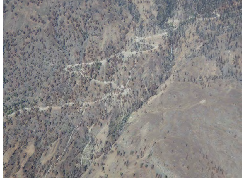
Photo 4: View of the Crater FSR with numerous drainage-related washouts and failures into Red Bridge Creek.
