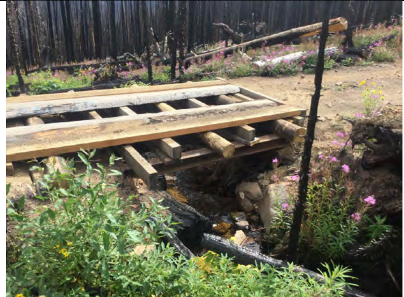
Photo 6: Scout Creek temporary bridge crossing along Lakeview Road (at ~12.5 km). One of two small bridge structures lost in the fire.
