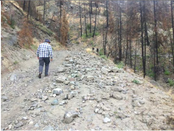
Photo 5: Washout along Crater Creek FSR at Red Bridge Creek.
