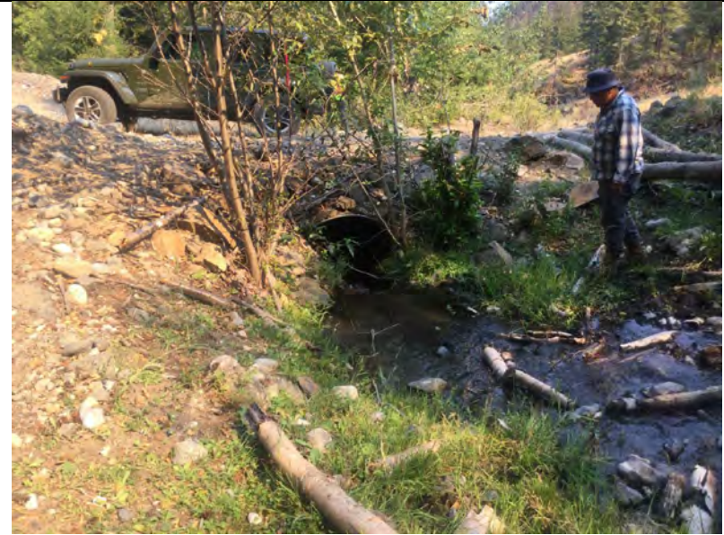
Photo 6: Culvert (1000 mm) inlet at Rattlesnake Creek crossing along Paul Creek Road. Outlet is partially obstructed by road grading sediment.
